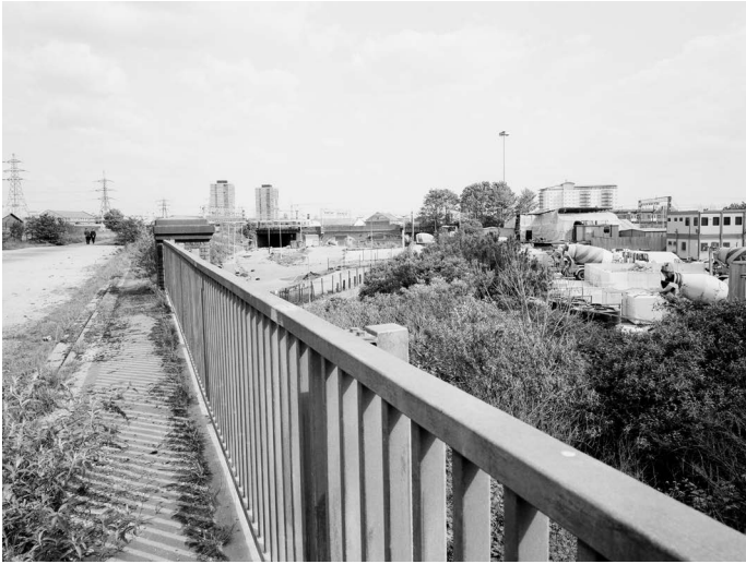
The Northern Outfall Sewer, 2003
