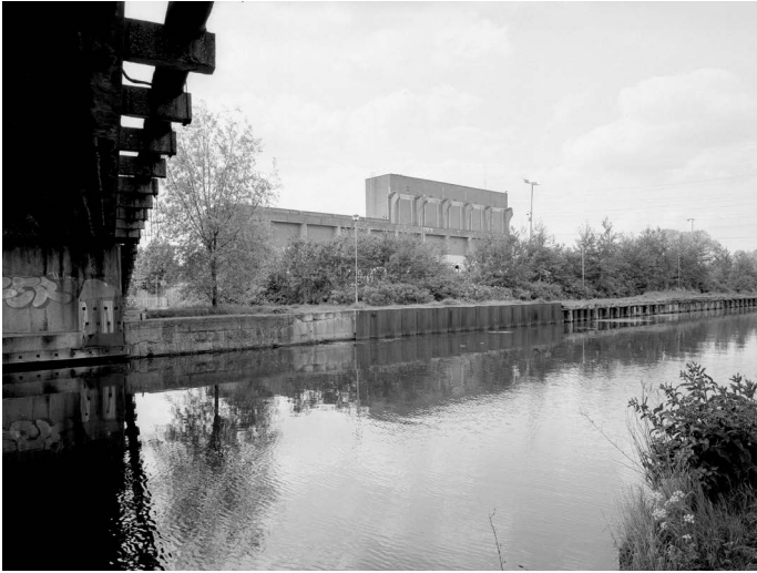
The remains of Lea Bridge Power Station, 2003
