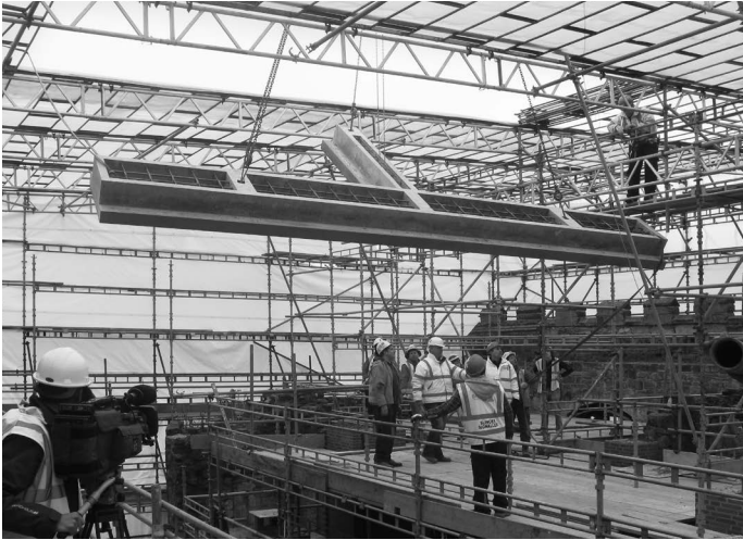
Astley Castle, lowering the hollow concrete "T" lintel into place
