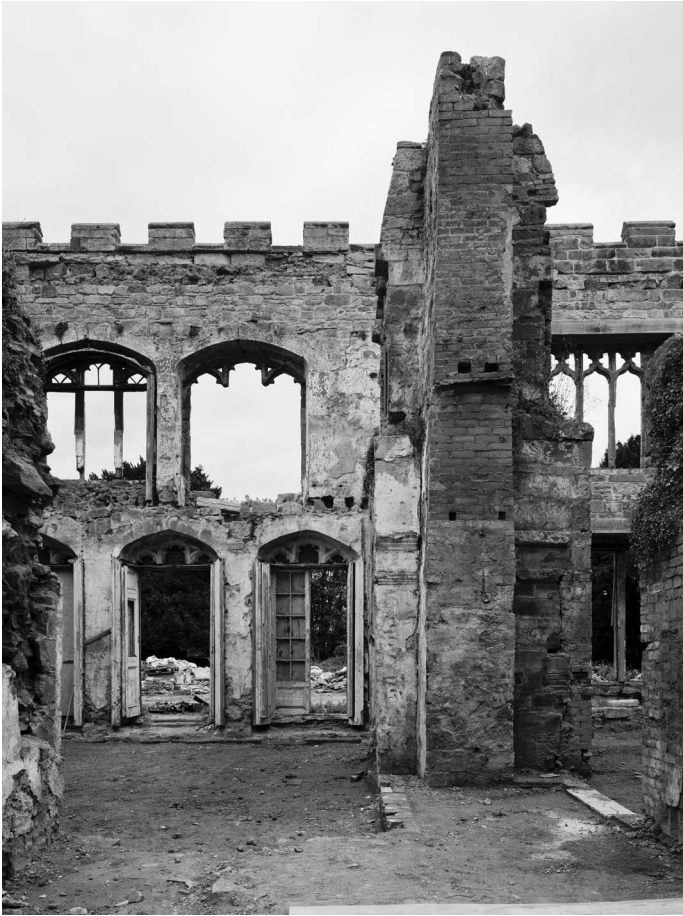
The ruin after clearance of rubble and other debris
