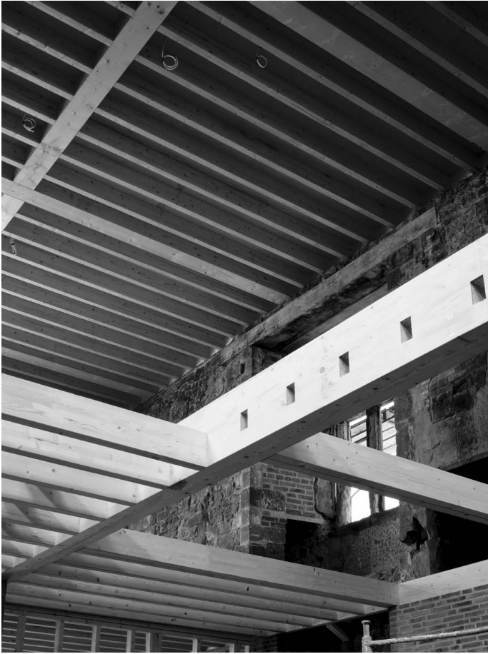
Roof and first floor in laminated timber, under construction
